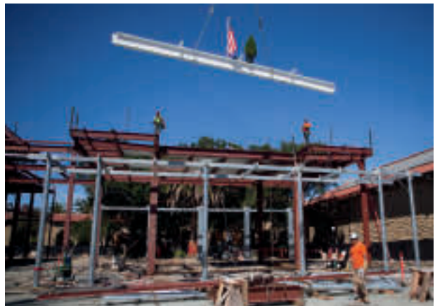
After the signing, construction crews lifted the 1,500-pound beam into place, carrying with it a traditional tree and American flag. PHOTO: DON FERIA
