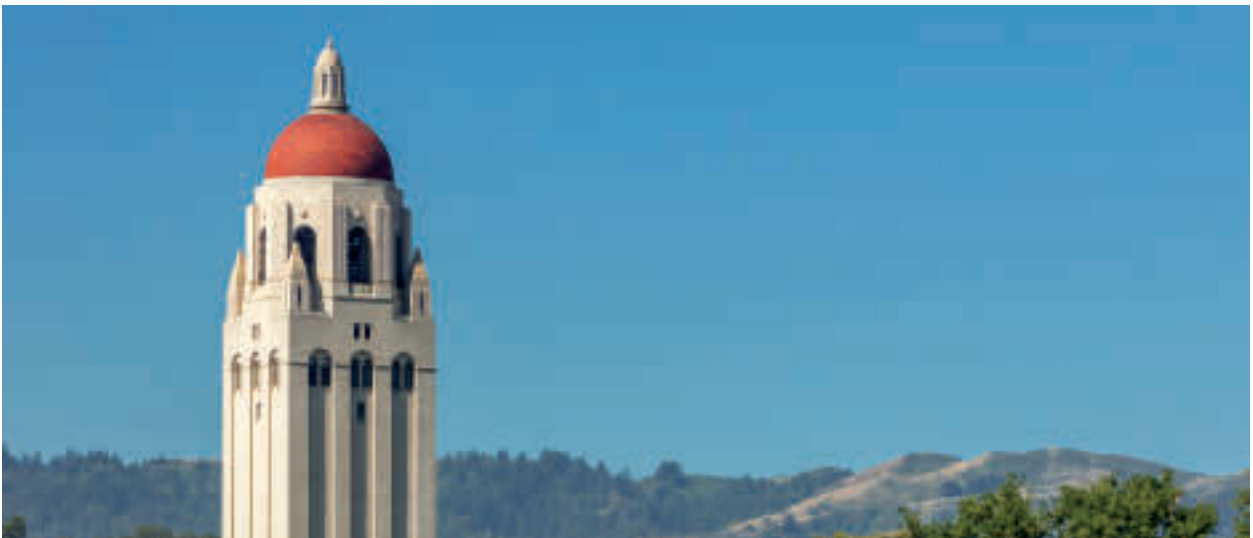
PHOTO: TIM GRIFFITH
