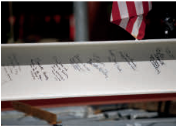
Lead project donors and other Hoover supporters attended a “topping out” ceremony for the David and Joan Traitel Building, signing the final steel I-beam before its installation. PHOTO: DON FERIA
