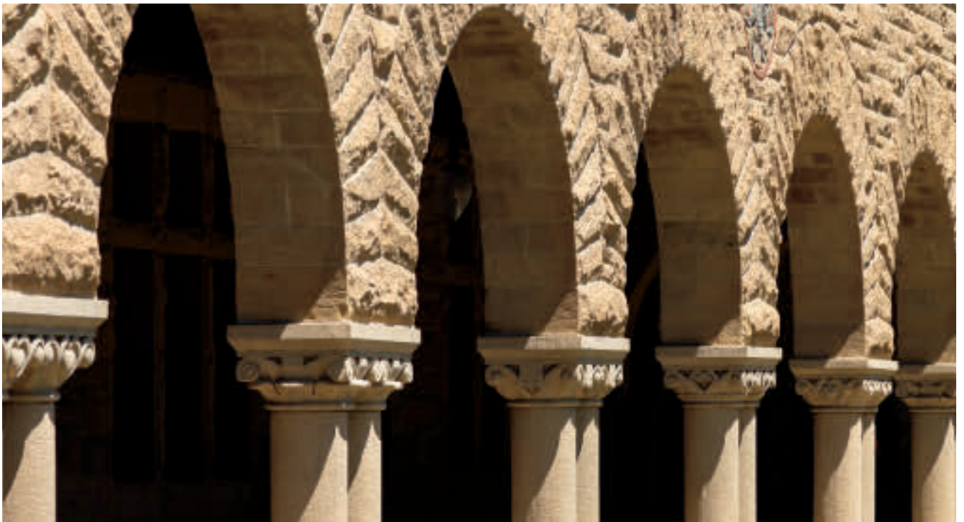
PHOTO: TIM GRIFFITH
