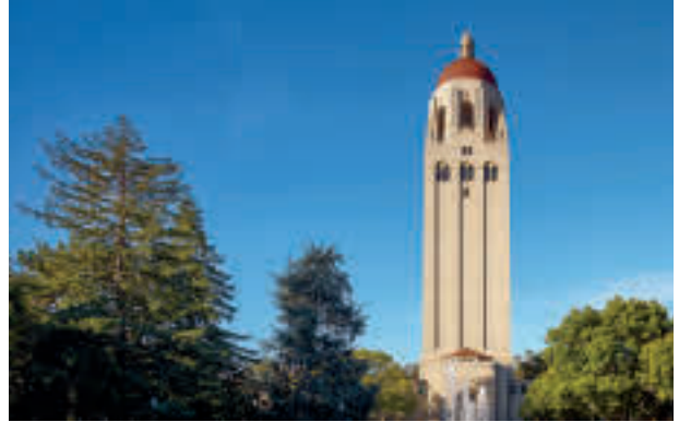
PHOTO: TIM GRIFFITH
