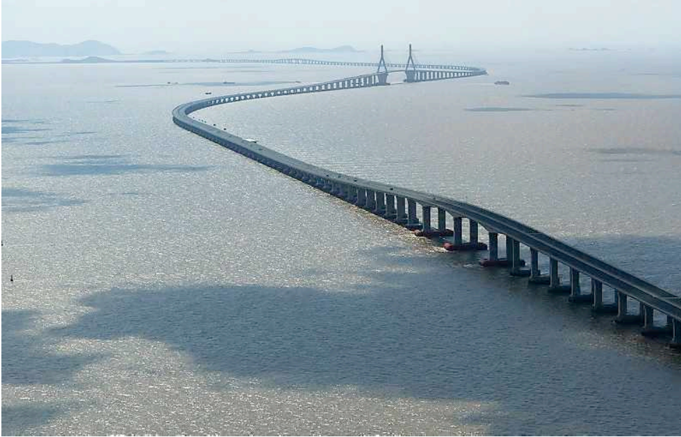
The East Sea Grand Bridge
