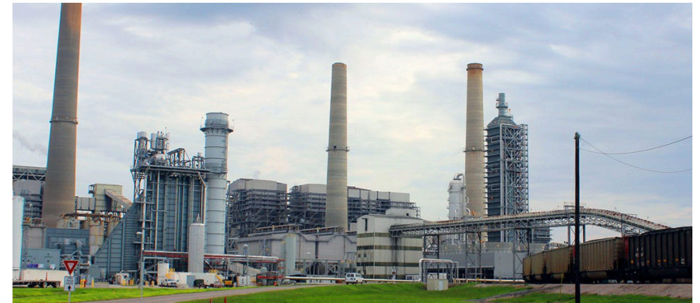
Petra Nova 240 MW coal-fired generation with post combustion capture: 1.4 Mt CO 2 /year .
