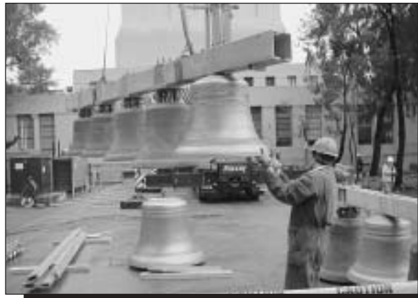
The carillon's 48 bells being lifted in groups to the Hoover Tower observation deck.
